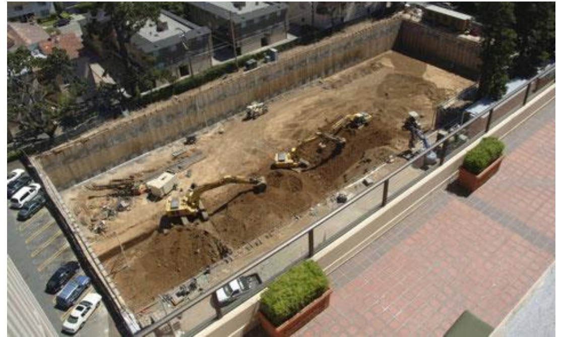
Typical Representation of Support of Excavation (SOE)
