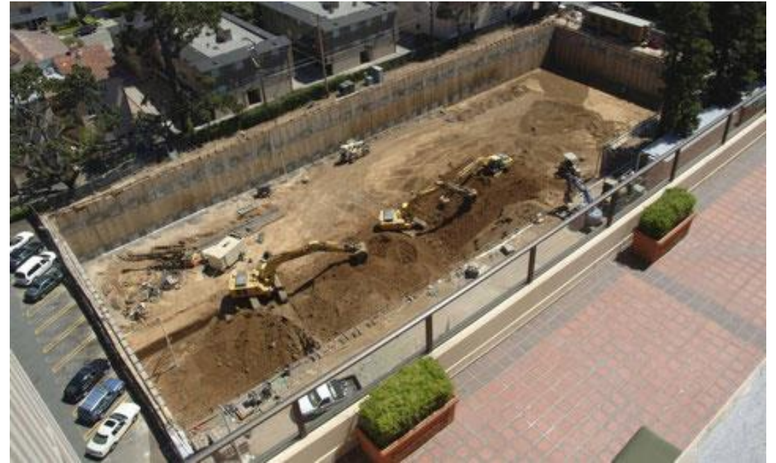
Typical Representation of Support of Excavation (SOE)
